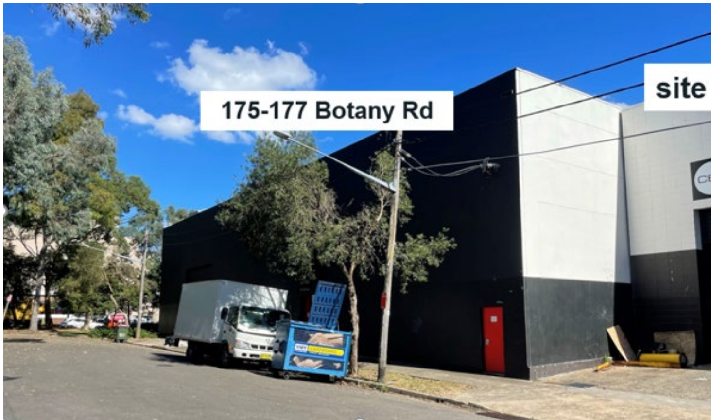
15 commercial development to south - 175-177 Botany Road – viewed from Cope Street
