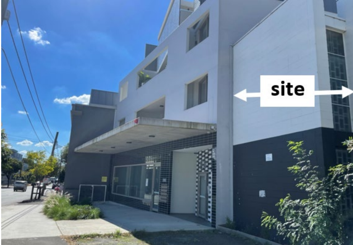
adjoining residential development to north - 169 Botany Road
